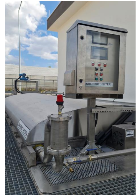
Custom Enrodisc Design for IPA Project, 1000 cubic meter per hour secondary effluent filtering.
