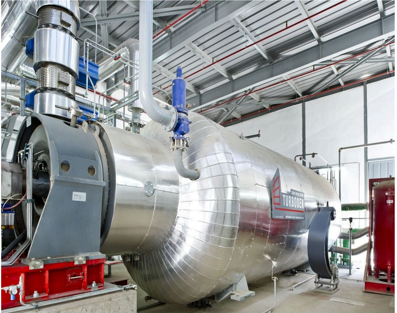
Figure 5. ORC Turbine & Generator
